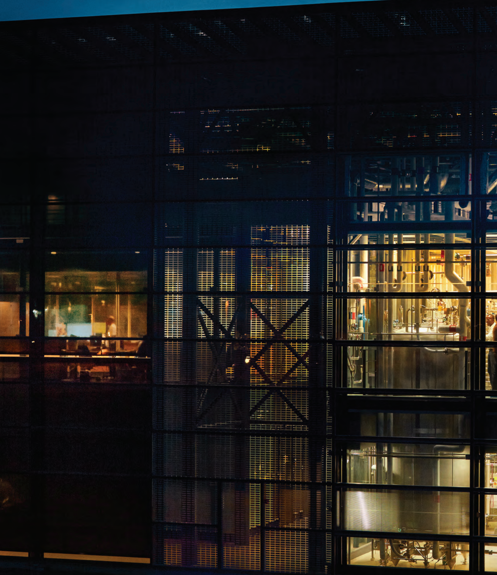
Novo Nordisk A/S, Hillerød, Denmark. Facility finished in 18 months for the life saving drug NovoSeven®.
