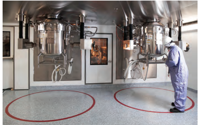
Centrifuge suite with two paste collection vessels containing the centrifuge bowls.
