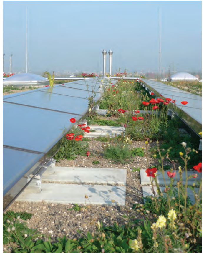
Solar panels on the green roof.
