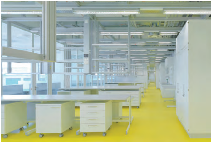
Open ceiling infrastructure in standard lab.
