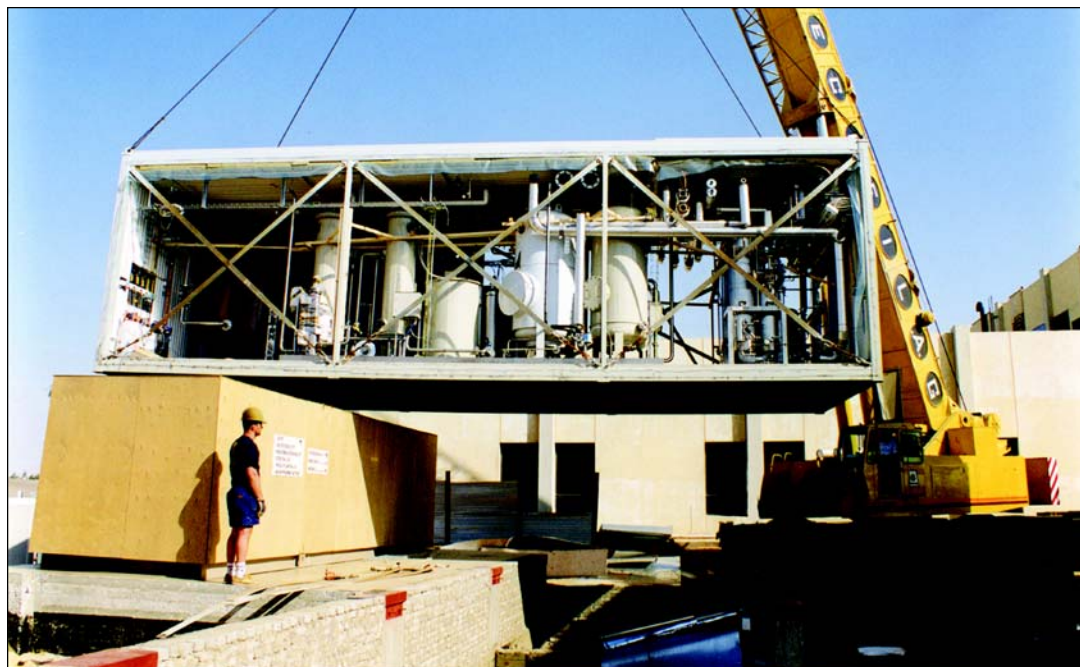
Figure 1. Typical standard facility module; external dimensions of 44'Lx15'Wx14'H (13.3x4.4x4.2M) with a floor area of 650F 2 (60M) and an average weight of 50 tons (cross-bracing shown for shipping purposes).
