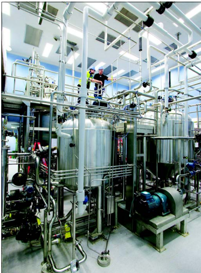
Figure 6. Final touches are applied after 12 months of field assembly.
