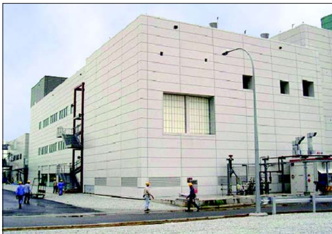
Figure 2. Relief panels in a modular facility with a stucco exterior that matches adjacent building.
