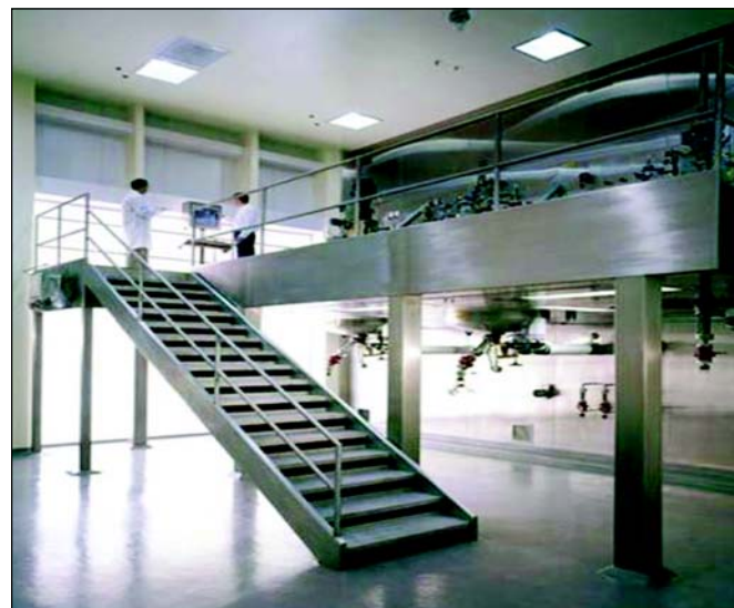
Figure 9. Modular unit installed and in operation. 11
